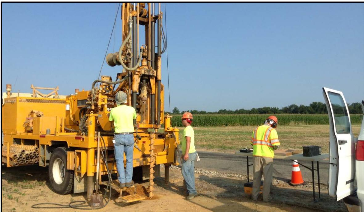
Figure 1. Typical STATEMAP drill site setup. Split spoon cores are collected, described, catalogued, and housed at the DGS for future reference and review.
